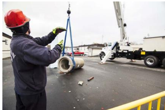
Gambar 58. Beban Crawler crane Terjatuh
