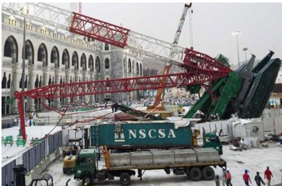
Gambar 57. Crawler crane Roboh
