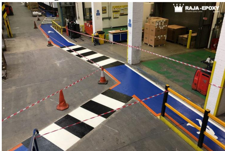
Gambar 6. 19 Marka area kerja (Sumber: https://www.raja-epoxy.com/wp-content/uploads/2018/08/pengecatan-garis-line-750x500.jpg )
