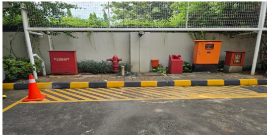
Gambar 65. Hidran halaman (I)
